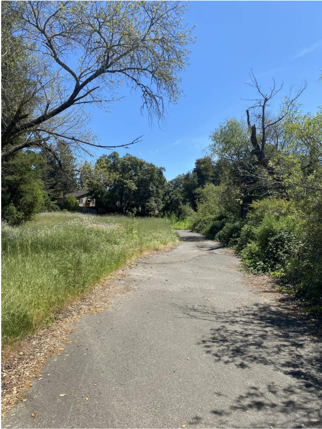
2 EXISTING ASPHALT DRIVEWAY (SOUTH)
