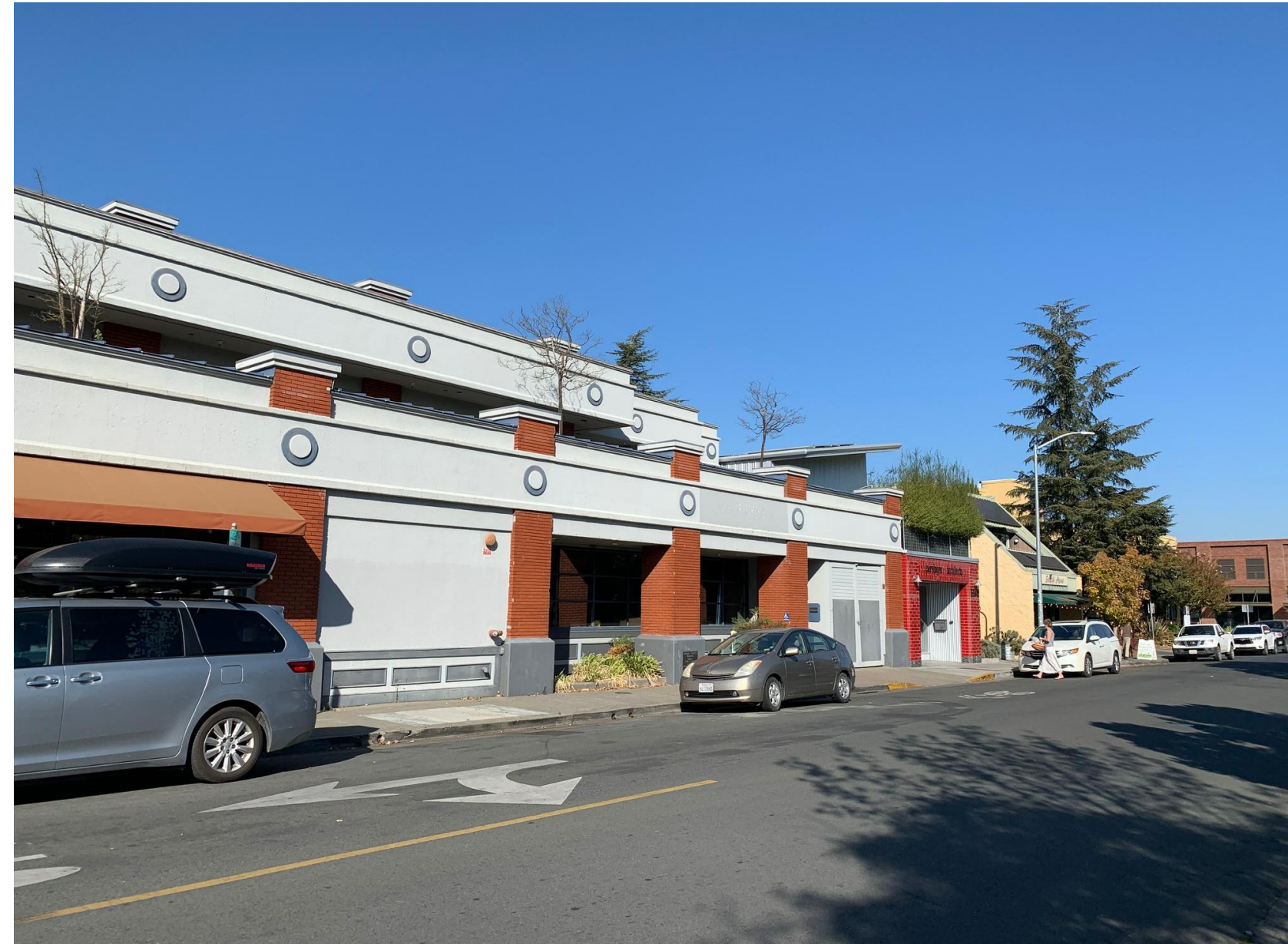
5 FROM BURNETT STREET LOOKING TOWARD EAST PETALUMA AVE.
