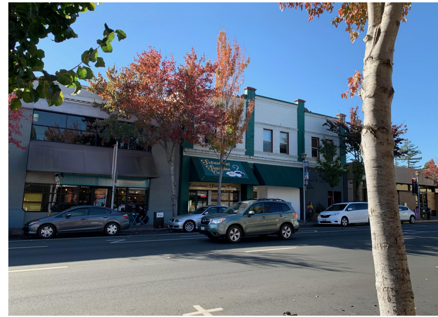
3 FROM PROJECT ENTRY LOOKING NORTH WEST ACROSS S. MAIN ST.
