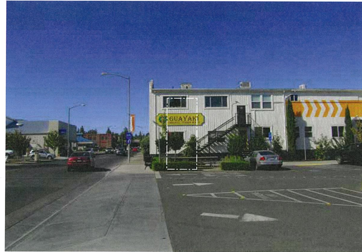
EXISTING CONDITION - WEST SIDE OF DRIVEWAY NOT TO SCALE
