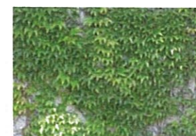
Vine covered CMU wall
