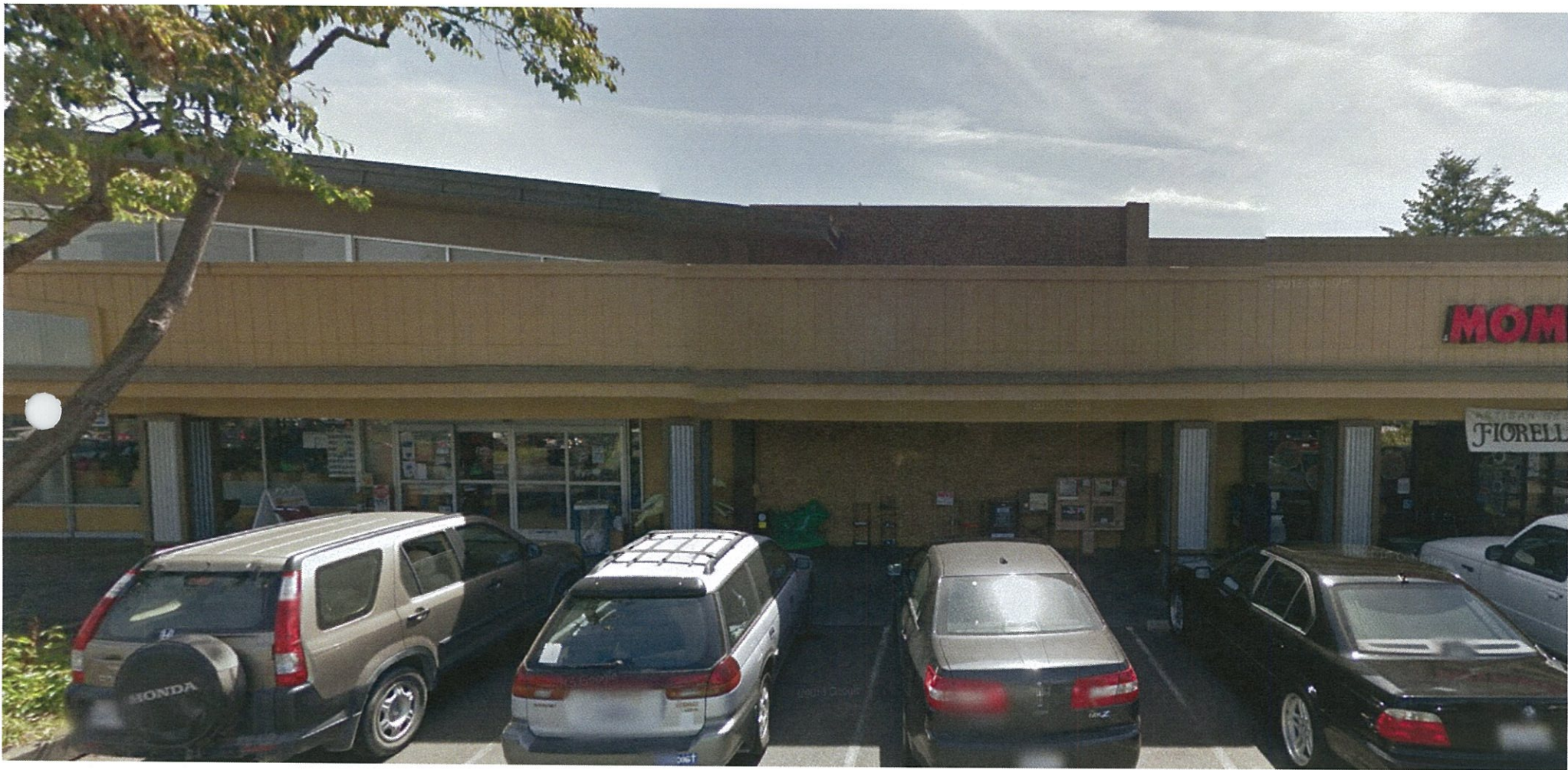
Existing 'Northern' section of the main entrance frontage proposed for the addition of corrugated metal.
