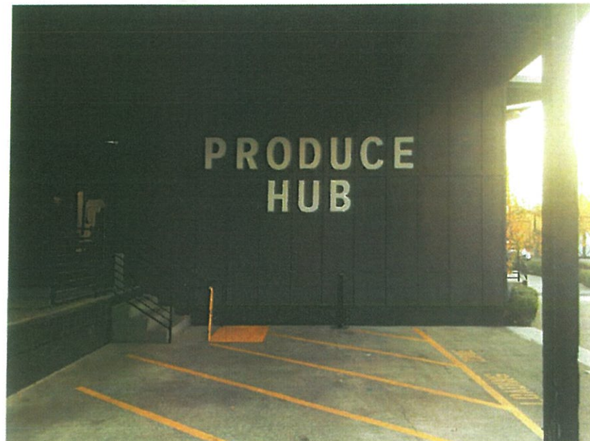
E-1 2 LOOKING SOUTH FROM LOADING ZONE, PHOTO #5 SEE. SHT E-3, DTL 1
