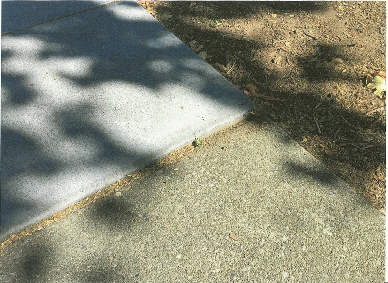
Sidewalk uplift from roots that has occurred since sidewalks were replaced
