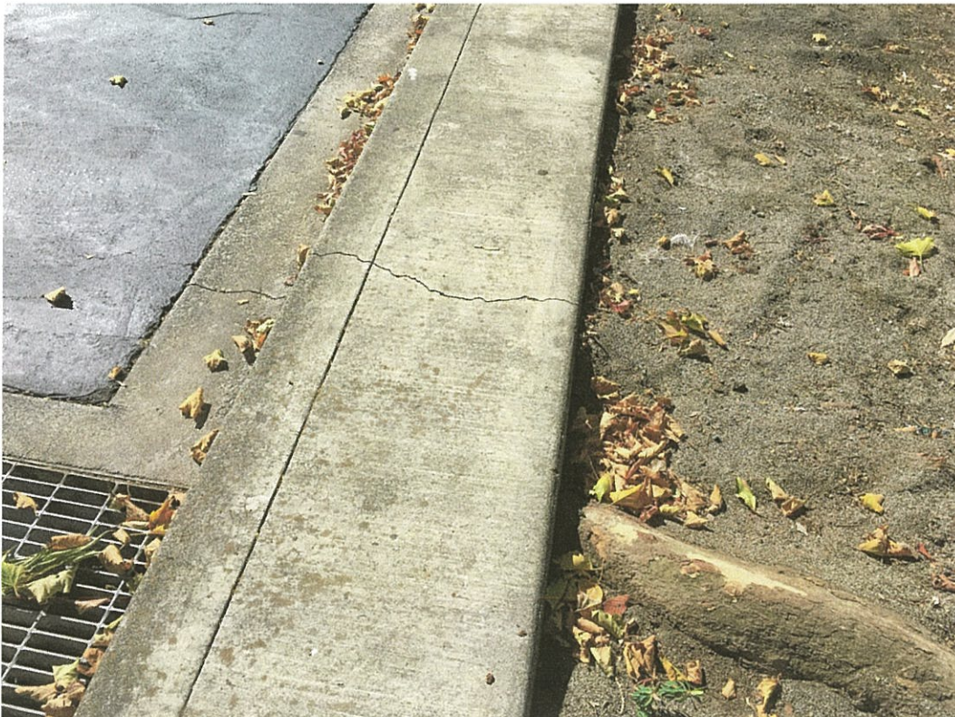
Large roots have left planting area and are uplifting surrounding concrete in search of water. These roots cannot be cut without damaging tree #2
