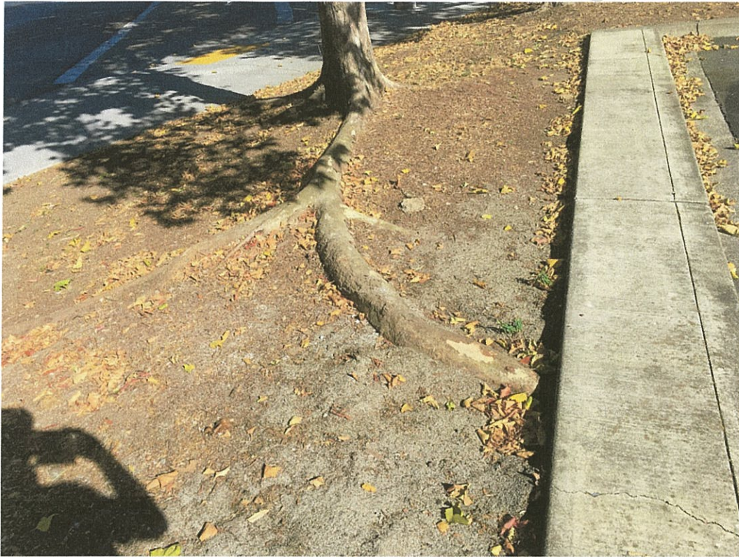
Large roots have left planting area and are uplifting surrounding concrete in search of water. These roots cannot be cut without damaging tree #1
