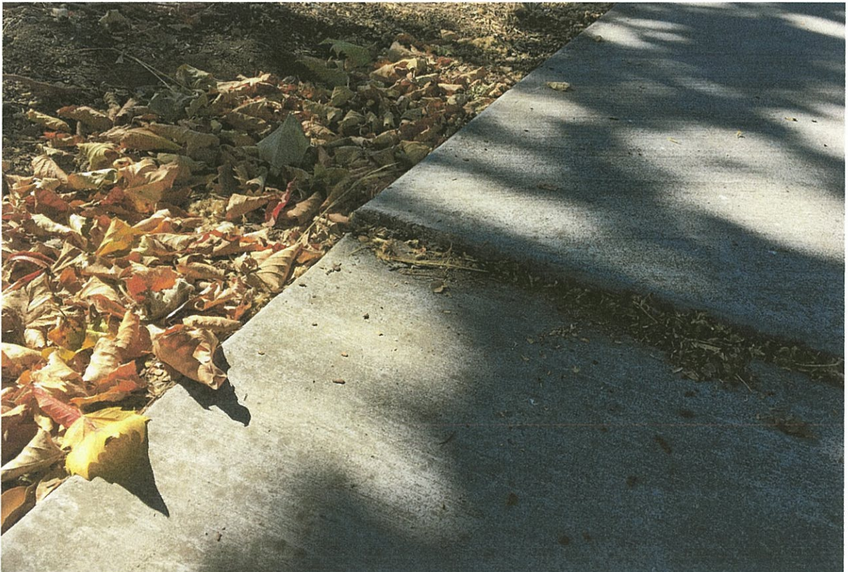
Sidewalk uplift from roots that has occurred since sidewalks were replaced
