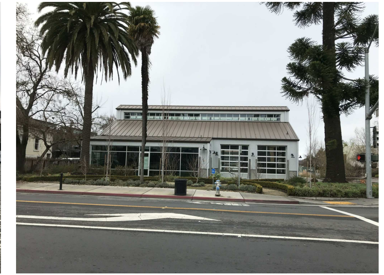
E SITE PHOTO E 12" = 1'-0"
