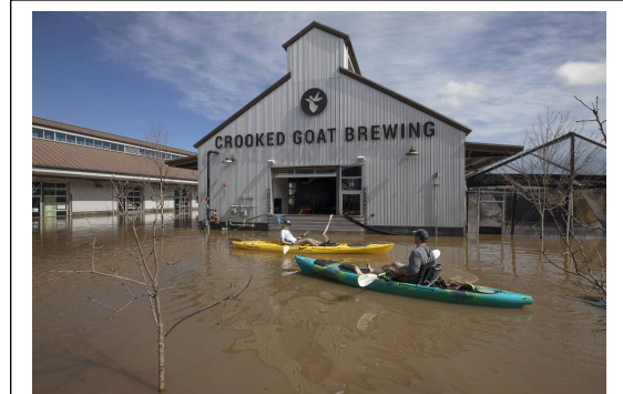
In February 2019, several businesses in The Barlow shopping district suffered from flooding after an atmospheric river stalled over the Russian River Watershed. An estimated two-thirds of the shopping district was flooded, including Park Village, a City-owned low income housing site, and the Community Cultural Center located on Morris Street. Photo Credit: John Burgess/The Press Democrat
