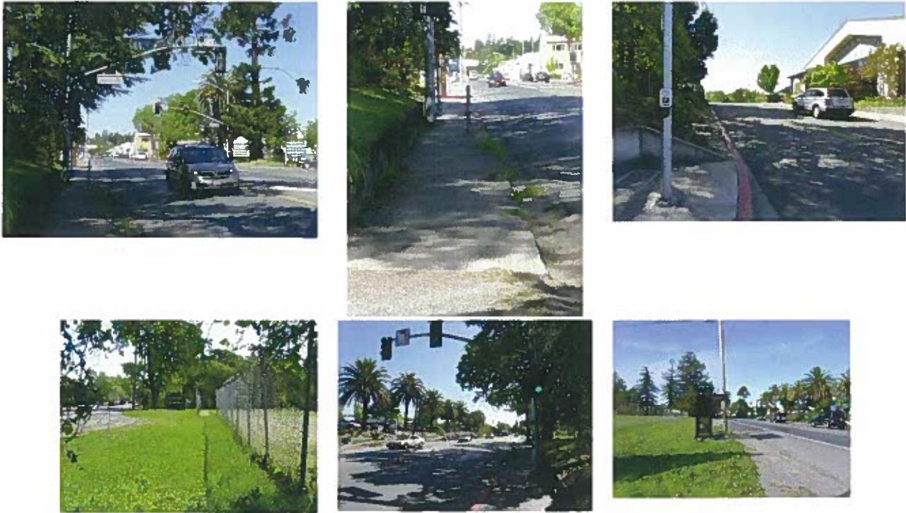
SEBASTOPOL AVENUE STREET FRONTAGE IS PLANNED TO BE RECONSTRUCTED BY CALTRANS WITH ELEVATED ROAD, SHOULDERS, SIDEWALKS AND NEW BUS SHELTER.
