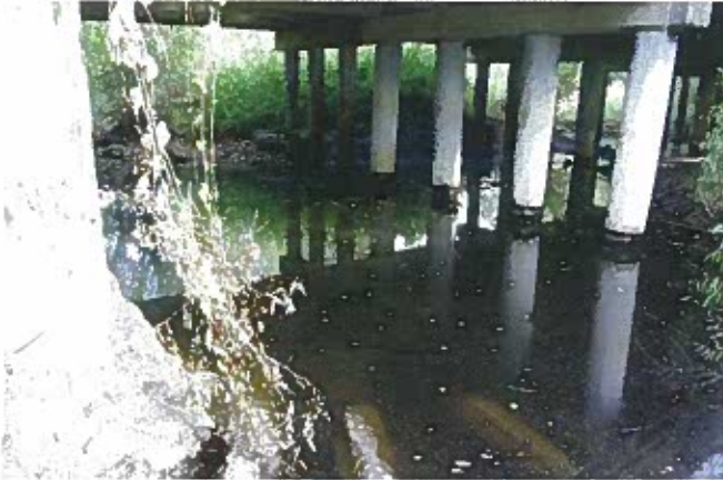
EXISTING SR 12 BRIDGE AT LAGUNA
