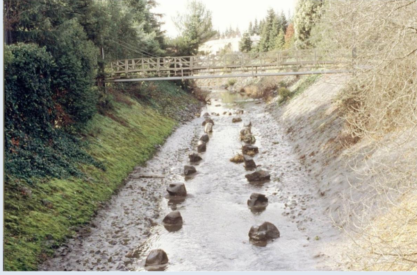
Santa Rosa Creek - Before
