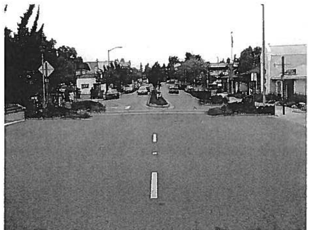
North Main Street at the post office. Pedestrians today attempt crossings while motorists are accelerating into place. Two future choices are available...if a one-way couplet is kept curb extensions are added. If a two-way street is adopted a median is also added.
