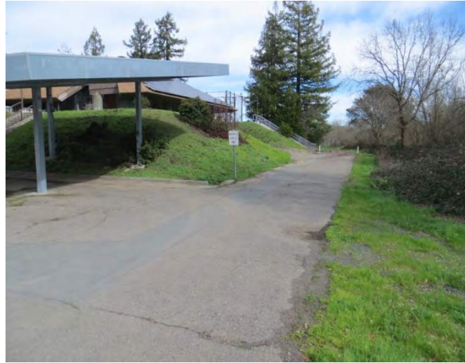
Access road to the wastewater lift station also serves as AmeriCorps Trail entry; adding entry signage will add visibility and welcome users.
