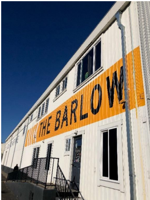
View of the western side of the existing building, looking north from SR-12.
