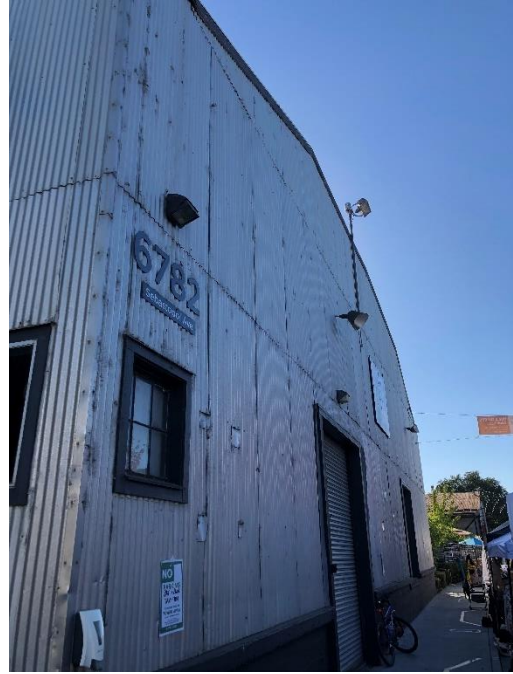
View of the northern side of the existing building, looking west from McKinley Street.
