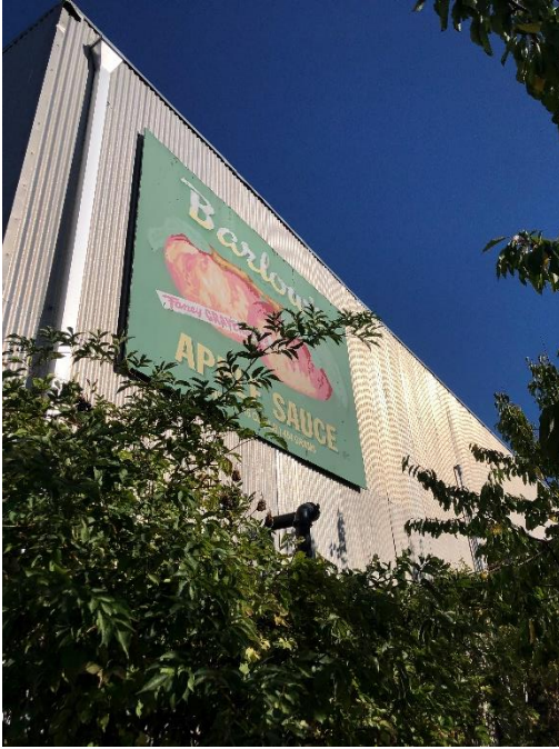
View of the northwestern corner of the existing building.
