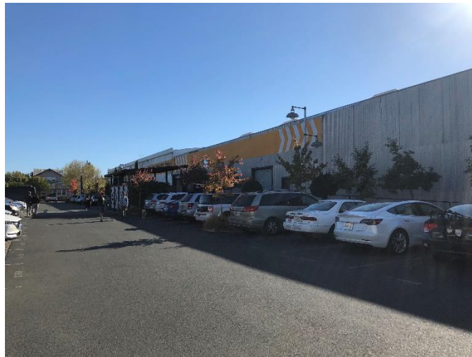
View of the eastern side of the existing building and parking area, looking south from McKinley Street.
