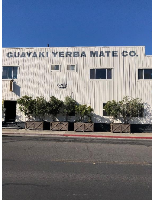
View of the southern side of the existing building, looking north from SR-12.
