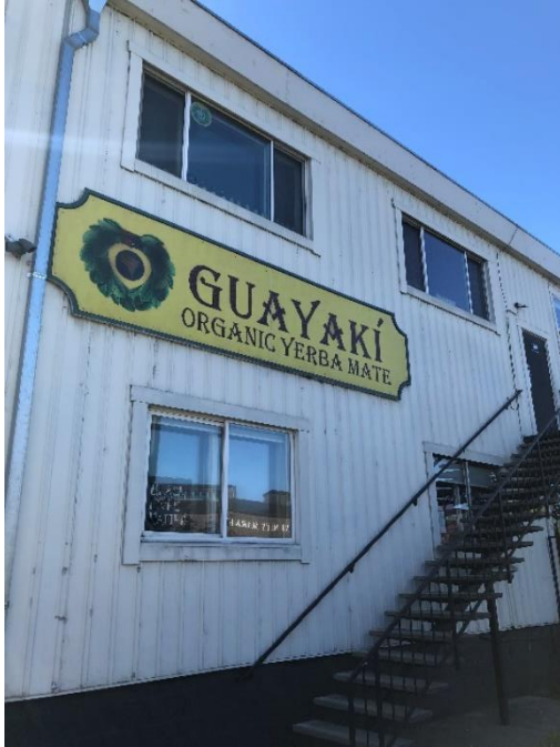
View of the southeastern corner of the existing building.
