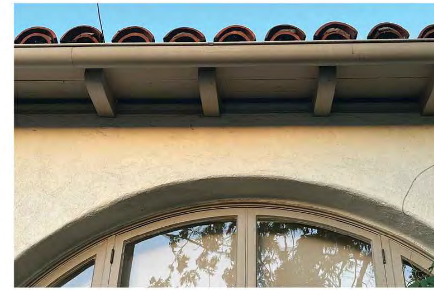
Painted Wood Rafters
